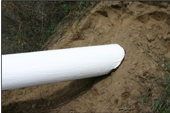
Prime Guard conditions the surface by displacing any moisture.
